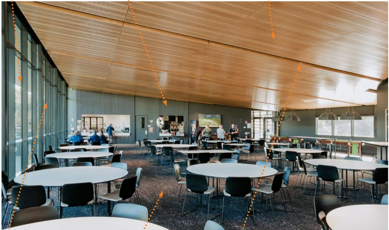
Full height front double glazed with aluminium powder coated framing system.
